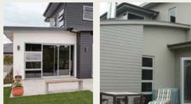
Plaster with Feature Cladding
